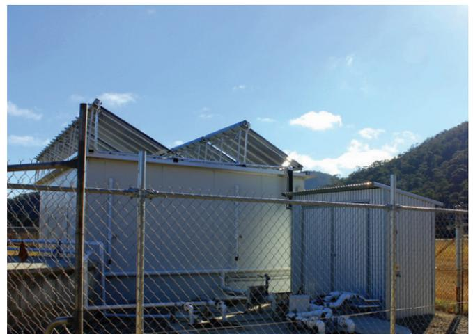
The insulated bio-chamber houses nine BioGill bioreactors.
